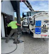
We are working on some service lines in alley A- B and having new stem risers built from Allstates machine out of Sugar City Idaho. This should help with the ability to turn these old service line valves. There are numerous water valves in Town that we cannot operate due to age.
